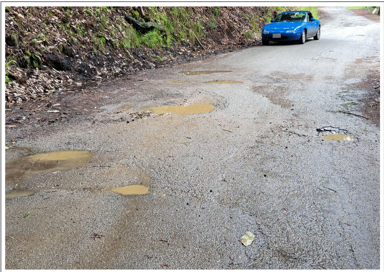
Figure 1. Laurel Road Pavement Condition Index (PCI) 10 in 2019 report. [1]
