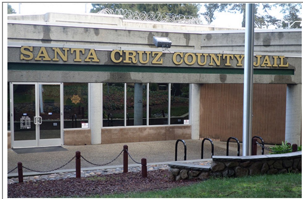
Figure 1: Santa Cruz County Main Jail. Photo courtesy of Ashley Keehn. [7]
