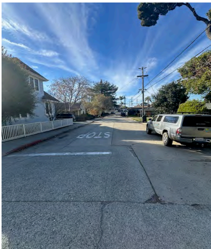
Photo 25: Inspection of 36-Inch Force Main (example of alignment route in service area (view 3))
