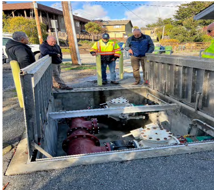
SITE E (Photo 2): Inspection force main valve box.
