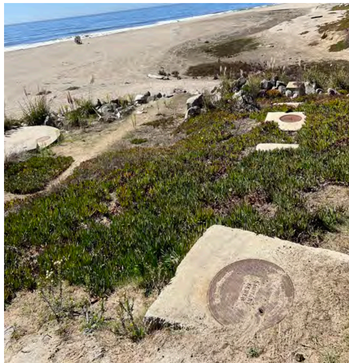
SITE B (Photo 6): View of maintenance manholes installed on beach looking west.
