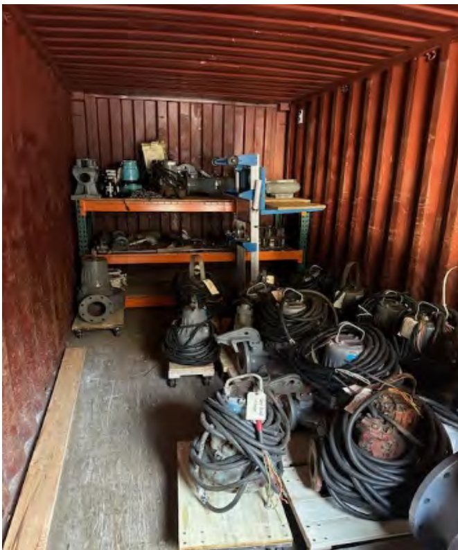
Photo 7: Corp Yard inspection (critical spare parts).
