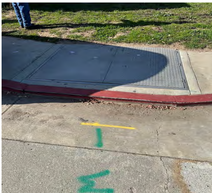
Photo 23: Inspection of 36-Inch Force Main (access to force main, inside is blind flange Tee that allows access into force main)
