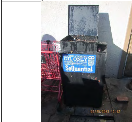
Photo 21: Used oil container near the grease interceptor of Capitola Diner, visible spill on ground.
