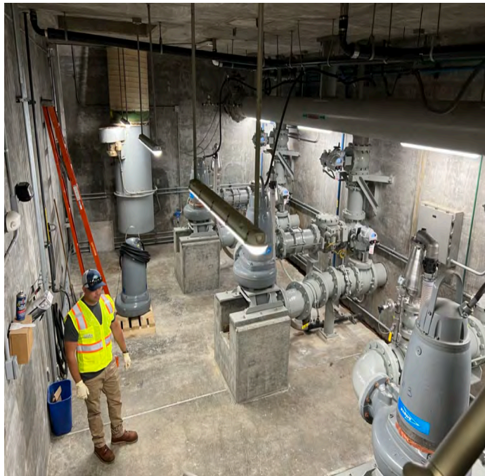
SITE B1 (Photo 14): Inspection of station dry well area; no "high water marks" observed on station walls in pit area.
