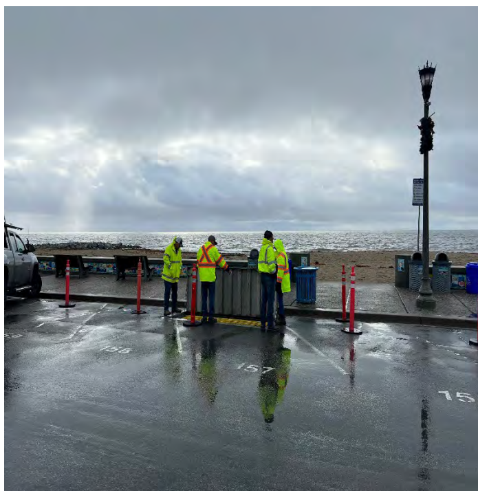
SITE B (Photo 3): Inspection of force main/bypass connection manifold in beach parking area (view 2).
