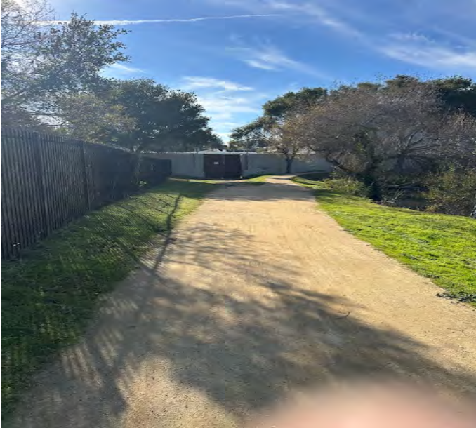
Photo 19: Inspection of 36-Inch Force Main (WWTP location where force main enters City of Santa Cruz Wastewater Treatment Plant at end of pipe)
