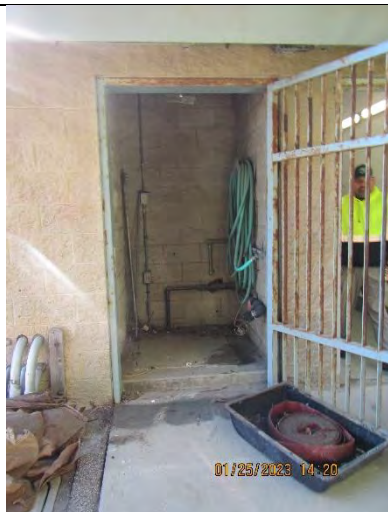
Photo 15: Wet well behind gate at Capitola Pump Station. Sandbags seen to the left used to protect wet well from recent storms.
