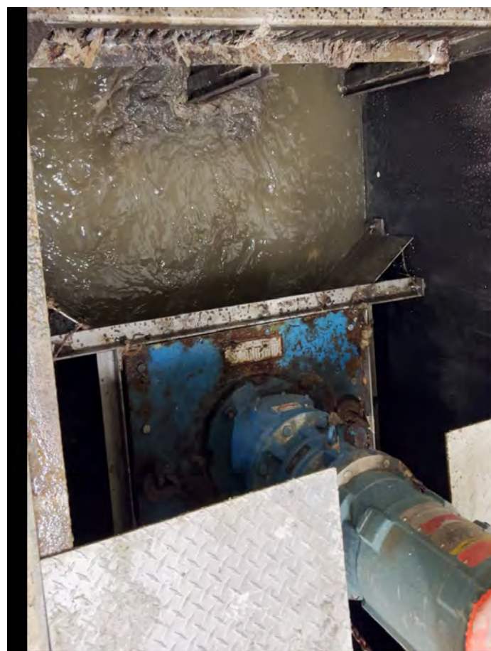
SITE D (Photo 4): Inspection of wet well.
