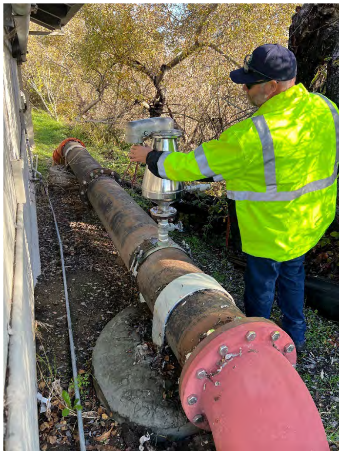
SITE E (Photo 3): Inspection of force main air release valve.
