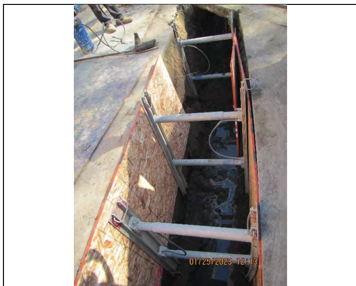
Photo 10: Open trench for the Rio Sands pipe replacement. Visible roots seen in trench.
