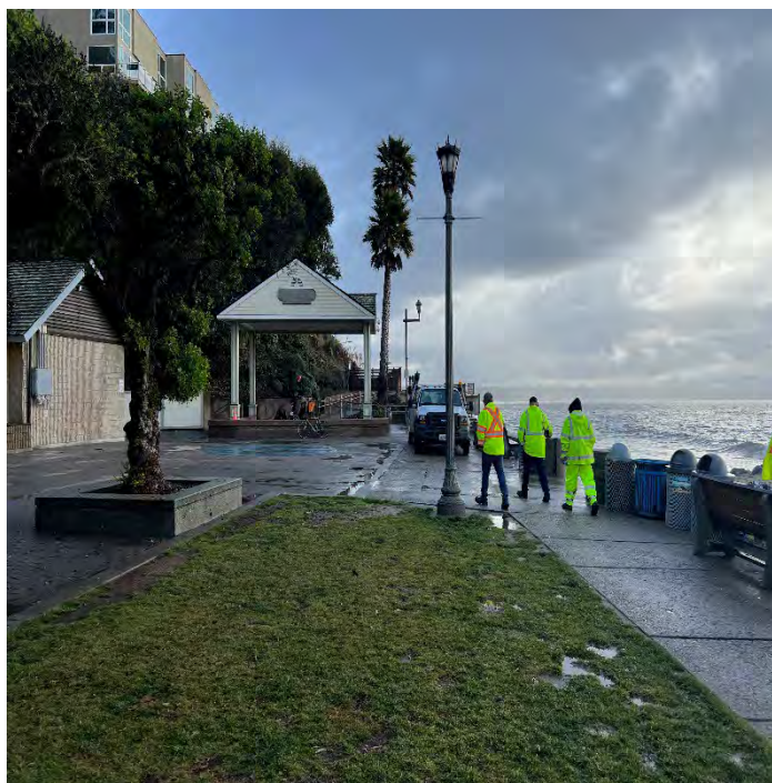
SITE B (Photo 1): View of entrance to Capitola Pump Station located approximately 100 feet from the Pacific Ocean.
