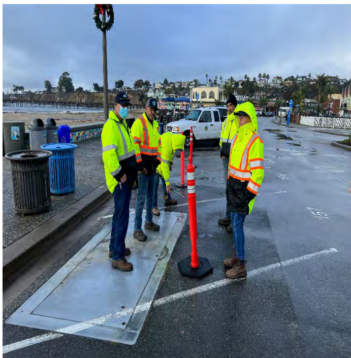
SITE B (Photo 2): Inspection of force main/bypass connection manifold in beach parking area (view 1).
