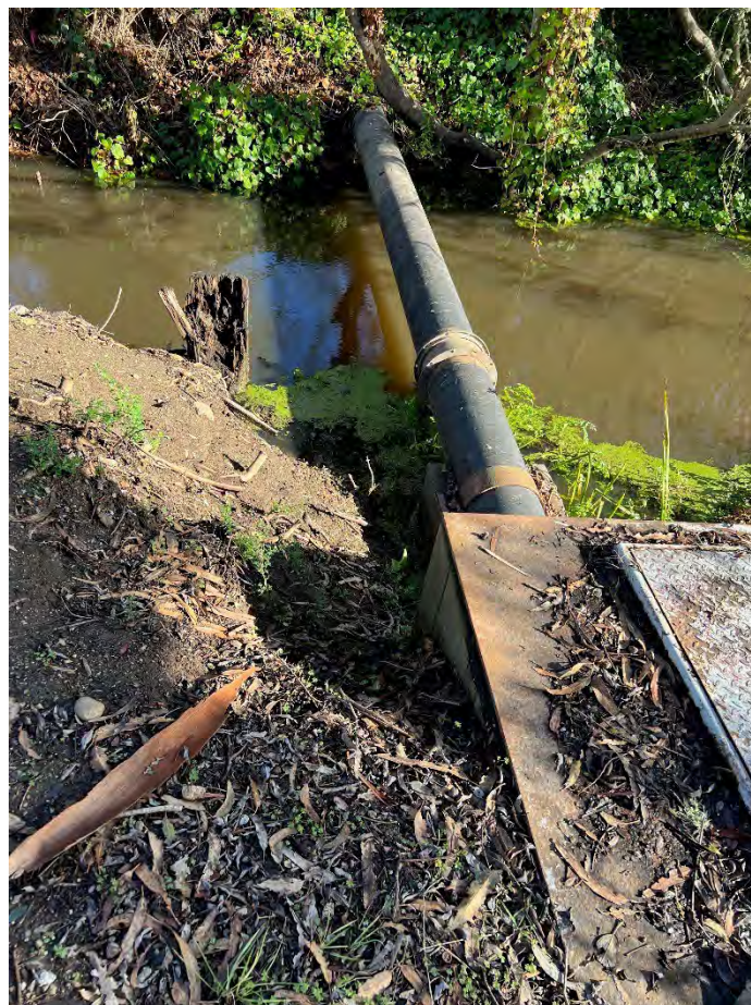
SITE E (Photo 4): Inspection of force main creek crossing.
