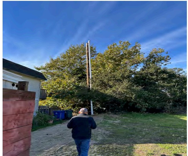
Photo 22: Inspection of 36-Inch Force Main (standpipe for odor control and highest point of force main)
