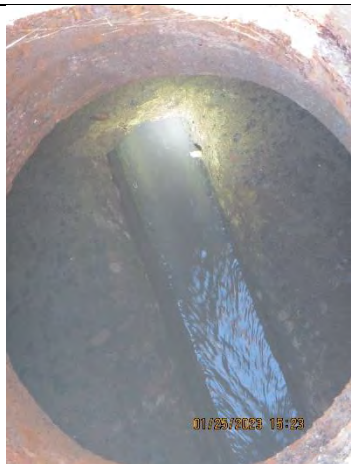
Photo 23: Manhole downstream of Capitola Diner with good flow and minimal FOG.
