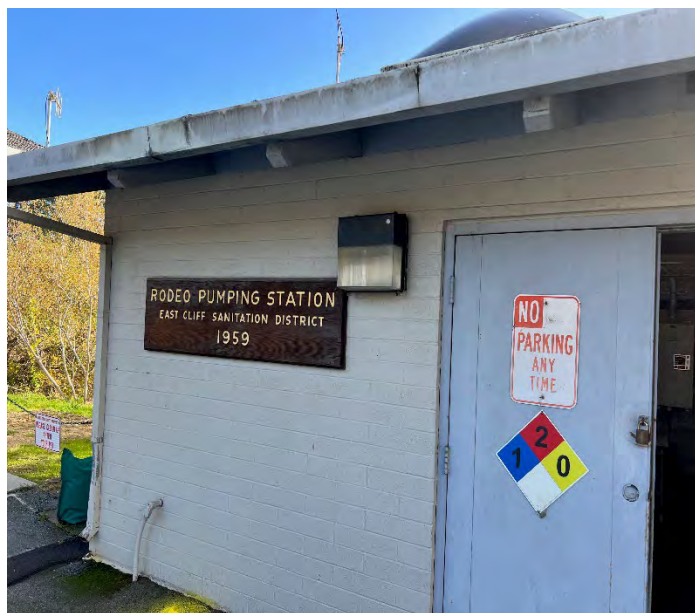
SITE E (Photo 1): Entrance to station with public signage.
