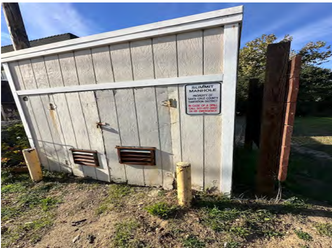
Photo 21: Inspection of 36-Inch Force Main (abandoned odor control facility)
