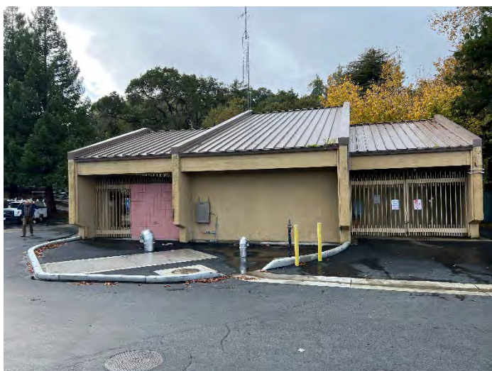
SITE D (Photo 1): View of pump station located adjacent to Peery Park/Soquel Creek in a large public shopping center.
