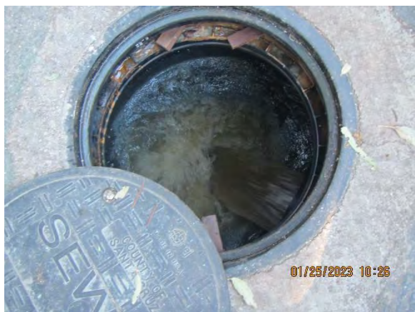
Photo 3: Manhole downstream of the Moran Pump Station leading to the D.A. Porath Pump Station with an observed high flow.
