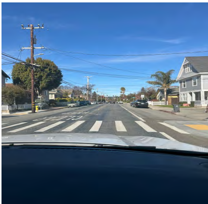
Photo 27: Inspection of 36-Inch Force Main (example of alignment route in service area (view 5))
