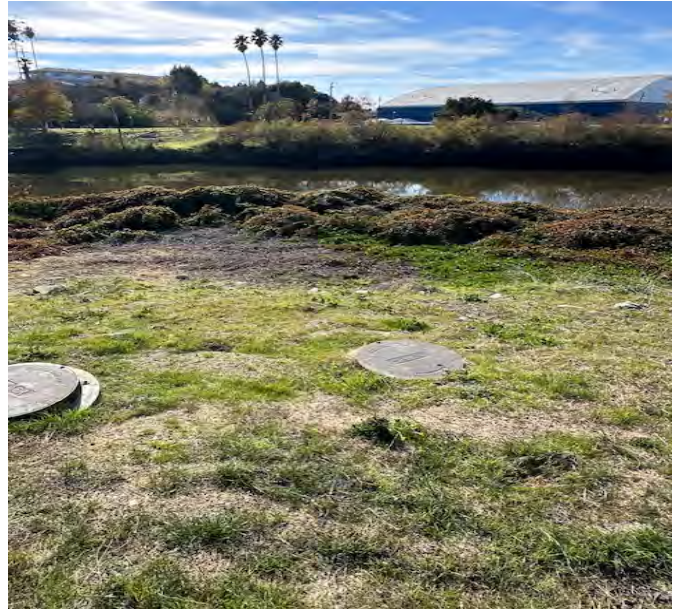
Photo 20: Inspection of 36-Inch Force Main (siphon location)
