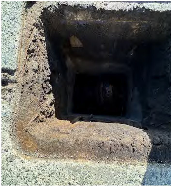
Photo 30: Inspection of 36-Inch Force Main (example of inside of typical valve box, with several of these located on force main route; according to operations staff, these valves have not been exercised in approximately 20 years)
