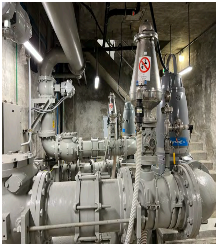
SITE B1 (Photo 16): Inspection of pumps/air release valves inside dry well.
