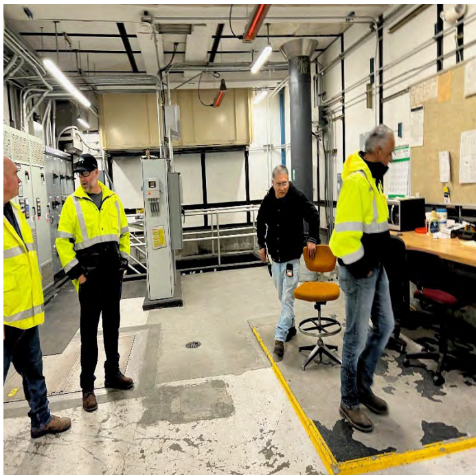
SITE D (Photo 7): View of station control room.
