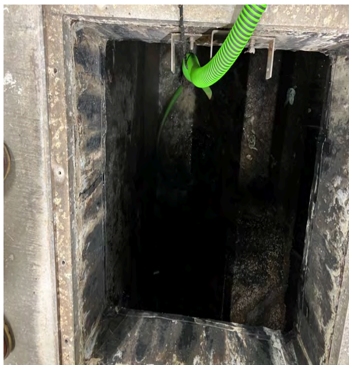
SITE B1 (Photo 17): Inspection of station wet well; no significant buildup of debris/grease observed.
