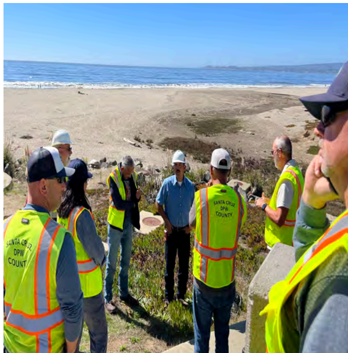
SITE B (Photo 3): Inspection of pump station looking west.
