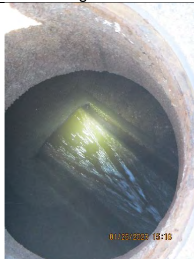
Photo 22: Manhole downstream of Capitola Diner with good flow and minimal FOG.
