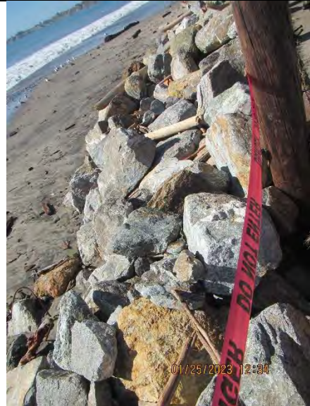
Photo 12: Rock barrier placed at the A1 Pump Station to protect the pump station from the storms.
