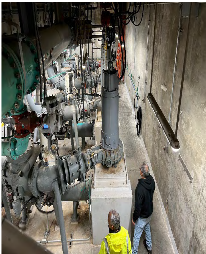
SITE D (Photo 5): Inspection of pumps/valves/force main.
