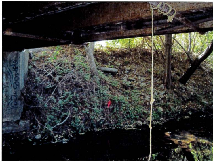
View of slope below bridge
