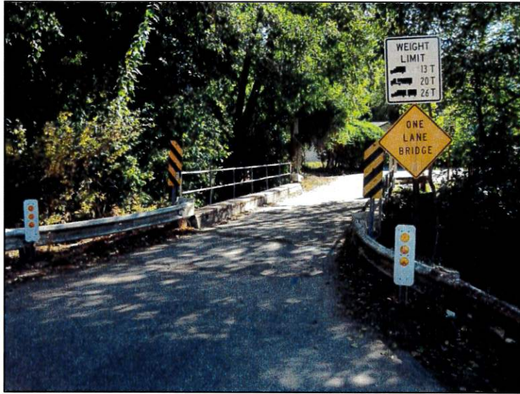
View of bridge, looking south
