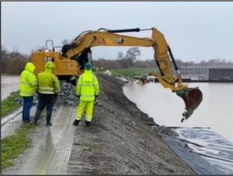
Left: Crews work to shore up part of the Pajaro River levee system. The Monterey County side would fail, flooding Pajaro.
